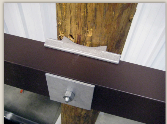
Top view of assembled PUPI EZE-Mount tangent crossarm assembly.
