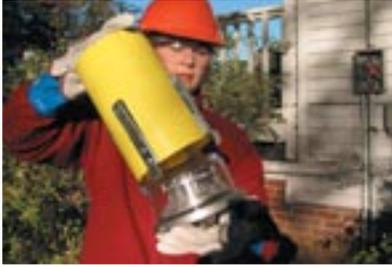
Insert meter into Meterpuller until locking clips snap onto meter's base.
