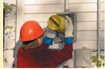
Depress locking clips to release meter and remove Meterpuller from installed meter.
