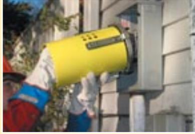
Align meter's contacts with socket and push meter into place.
