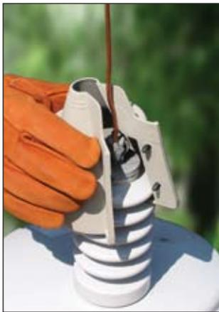
Rubber Glove Installation of R-21116
